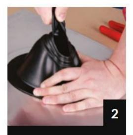
Finish adjustments to flashing opening by hand.
