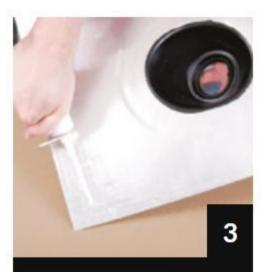
Apply sealant on the underneath of the metal base.
